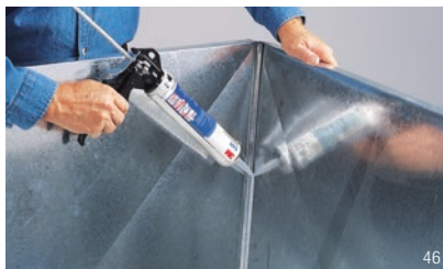
Seam sealing ductwork with 3M™ Polyurethane Sealant 540 will prevent air and dust intrusion. Its flexibility assists with vibration damping.
